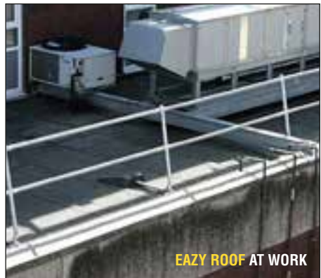
EAZY ROOF AT WORK
